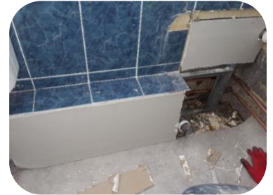
Replacing pipework inside boxing
