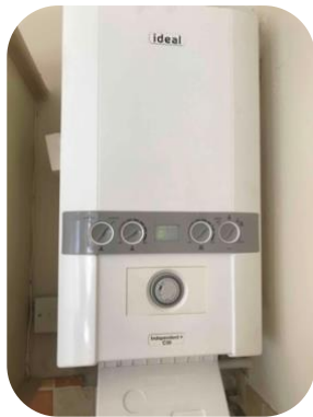
Installed new Ideal boiler
