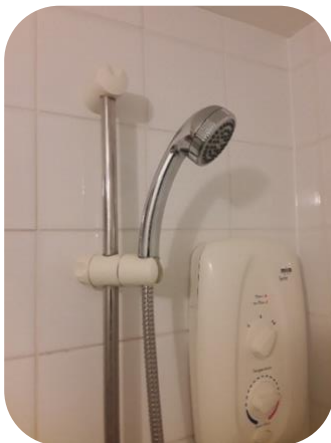
New shower installed
