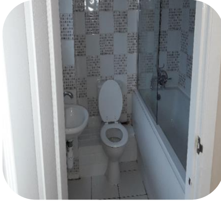
Installed new Full Bathroom
