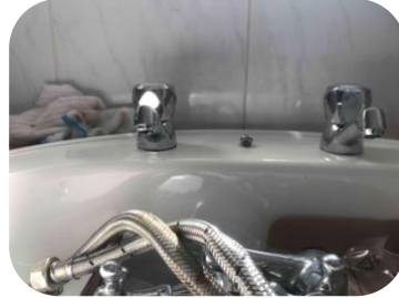
New mixer taps following replacement
