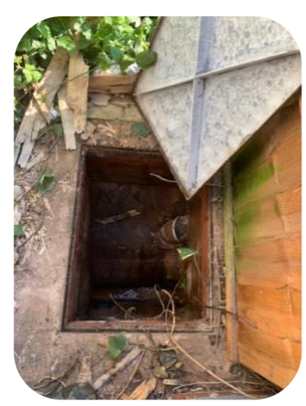
Inspected all the manholes around the property
