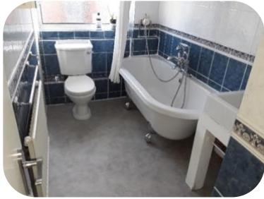
New bathtub toilet & sink installed
