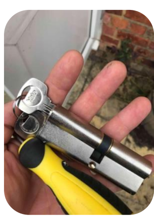
Installed new PVC door lock
