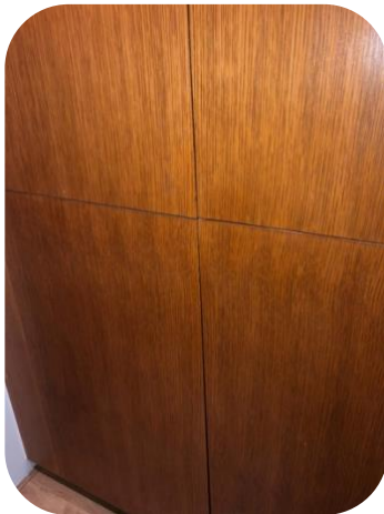
Adjusted & repaired fallen wardrobe
