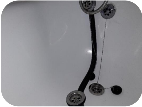
Replacing bath overflow waste pip
