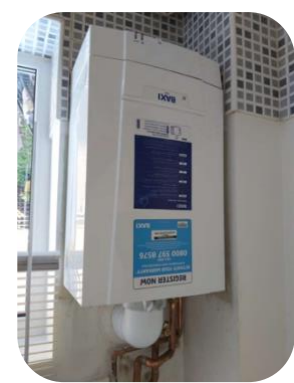
New boiler installed
