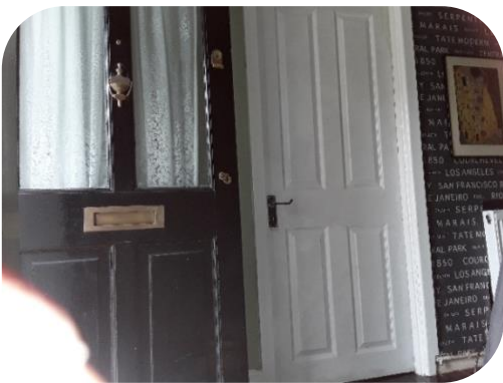
New fire door installed
