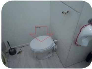
New toilet installed
