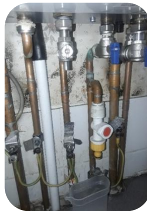
Installed new compression boiler valves
