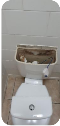
Replacing toilet flusher
