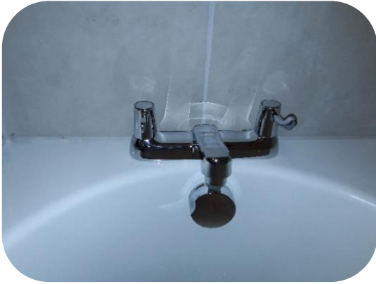
Installed new bath mixer taps
