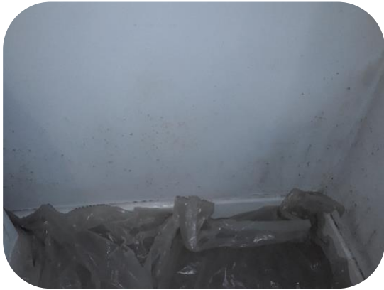
Dust sheet installed before painting
