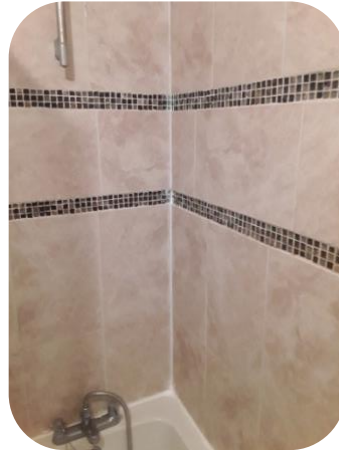
Grouted all bathroom tiles
