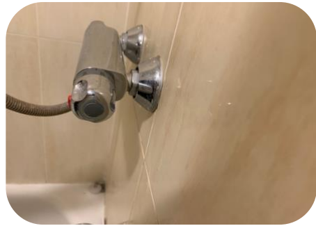
Tidy job, tiles were not damaged
