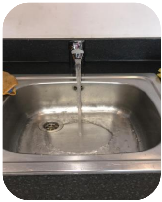
Installed new sink & mixer tap
