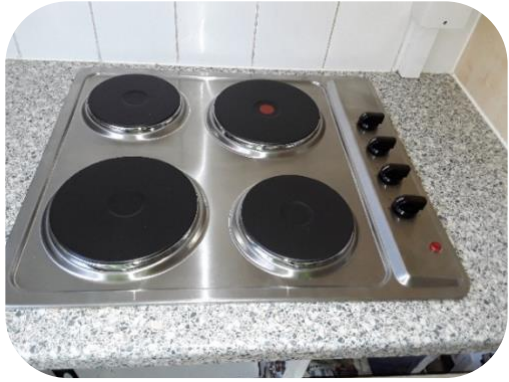
New electric hob installed
