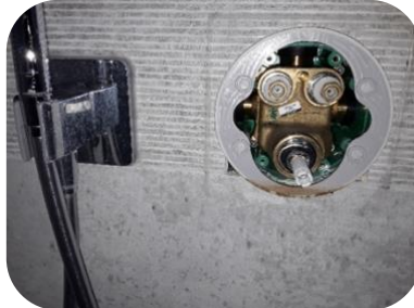
Installed new cartridge
