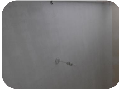
New ceiling following painting
