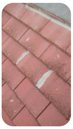
Damaged tiles replaced
