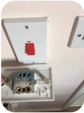
Isolation switch replaced
