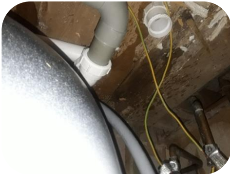
Installed bathtub waste pipes
