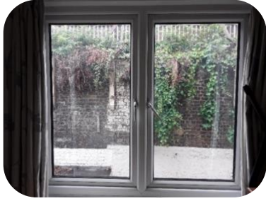
New PVC window installed
