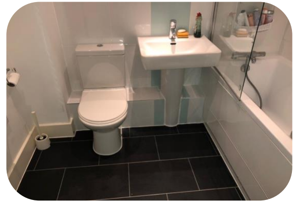
Pipework boxing (after)
