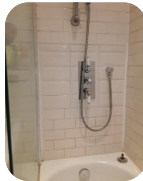
New tiles installed, grouted & made good
