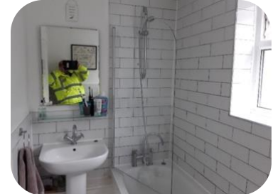
New bath screen installed
