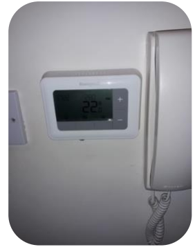
New room stat installed
