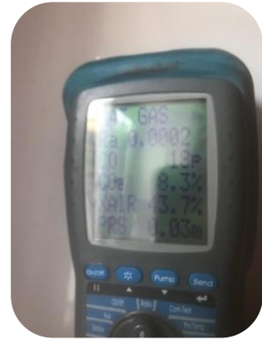
Flue test on new boiler
