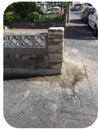
Repaired entrance wall
