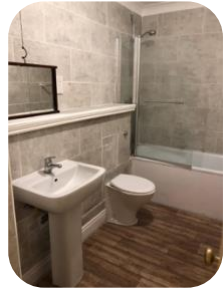
New bathroom, tiling & flooring installed
