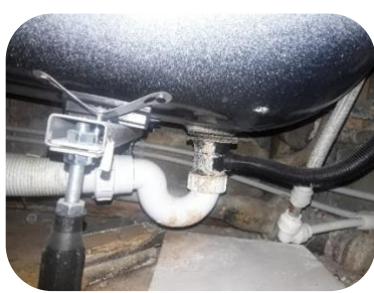
New trap installed under bathtub
