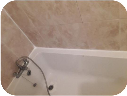
Applied silicon around bathtub
