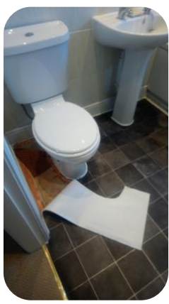
Installation of vinyl floor (before)
