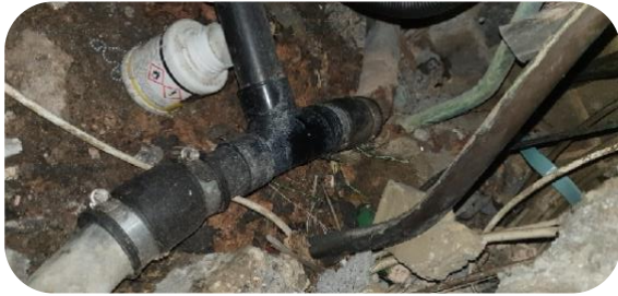
Repair to leaking joints under bath
