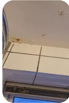
New tiles installed
