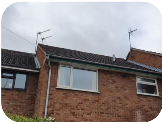
Installation of new gutters
