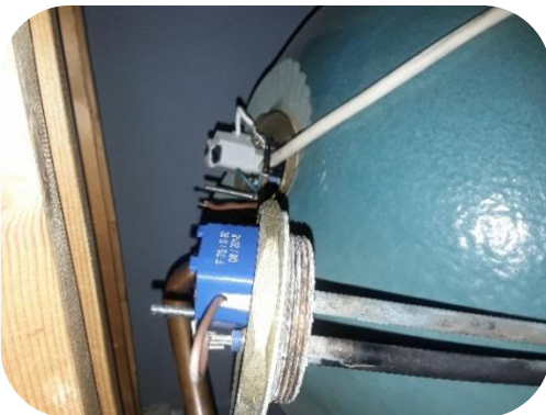
Old element being removed
