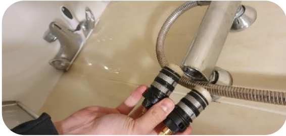
Replacing shower valves
