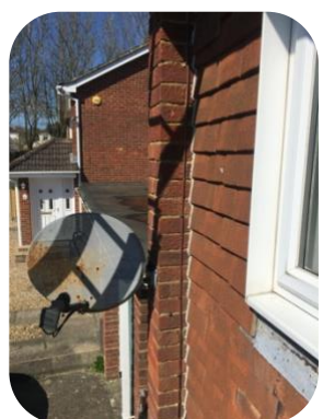
Repair to TV aerial
