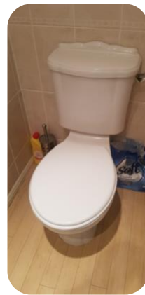
Supplied & installed new toilet & lino flooring
