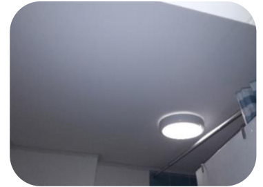
New ceiling installed
