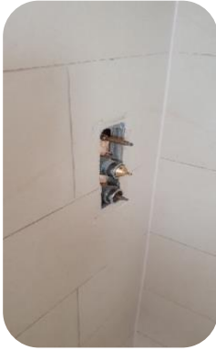
Installation of new shower cartridge
