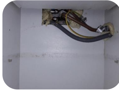
New earth bonding & WM inlet hose
