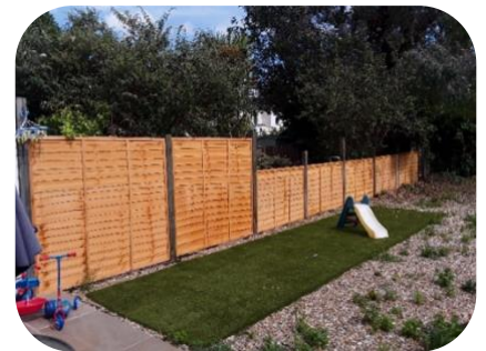
Garden left clean after fence installed
