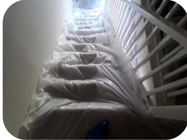
Covering carpets to prevent damage
