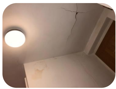
Damaged ceiling
