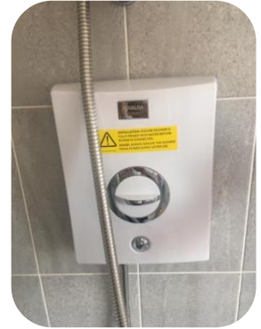
New electrical shower installed
