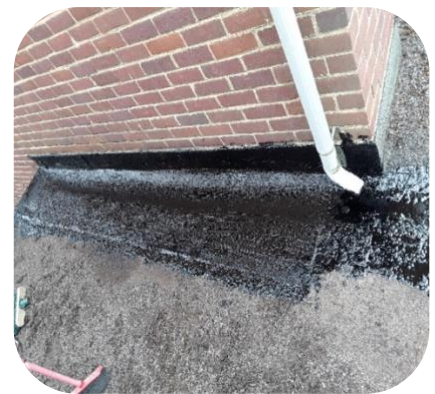
Repaired roof & reapplied roof tar
