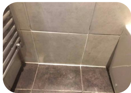
New grouts on tiles
