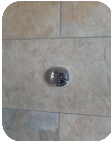
Shower thermostatic valve repaired
