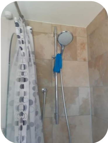
New shower handle railing installed
