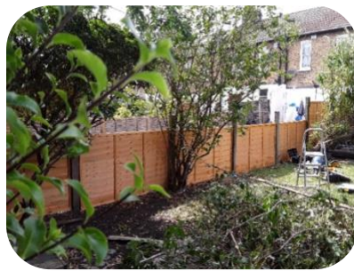
New fence installed
