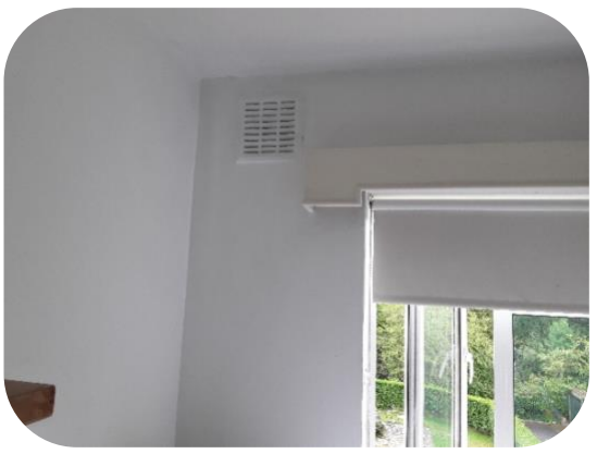
Painted living room after repairs to walls
