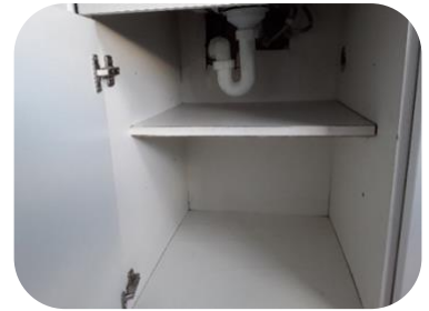
New under sink waste trap installed
