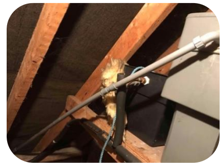
New cold-water tank overflow pipe installed
