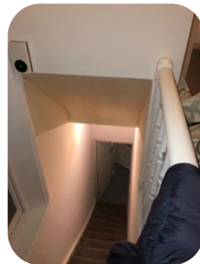
Installed new bannister
