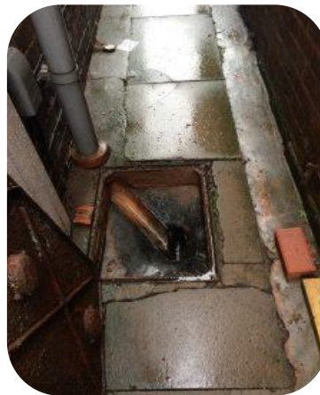
Unblocked manhole & tested water running
