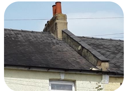
Full repointing of the roof
