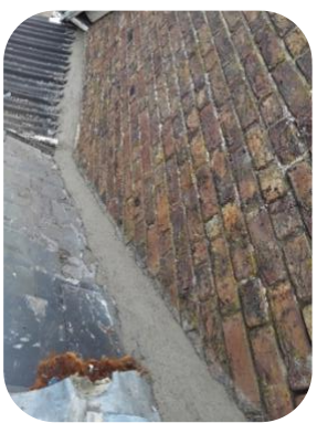
Sealed full roof hips
