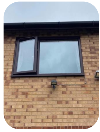
Installed new window
