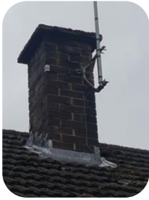
Chimney pointed & new lead flashing
