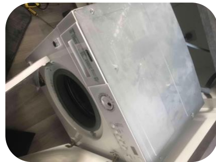
Washer & Dryer being installed
