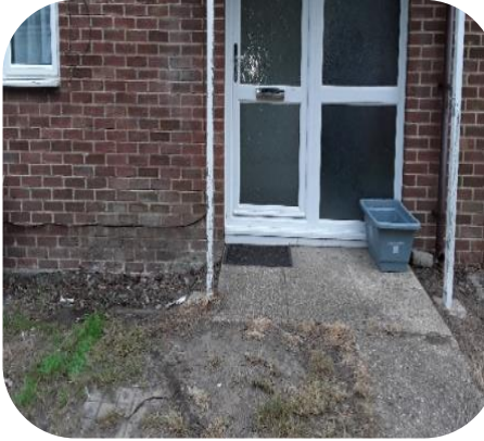
Installed new PVC Entrance door
