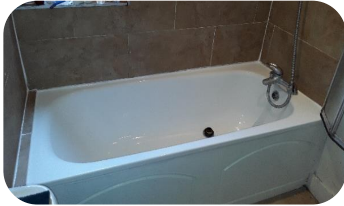
New bathtub & new tiles installed
