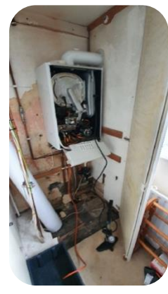
Testing boiler for safety following the work
