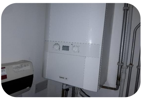
Installed new boiler
