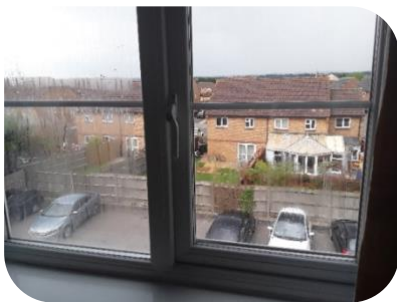
Adjusted & repaired the PVC window
