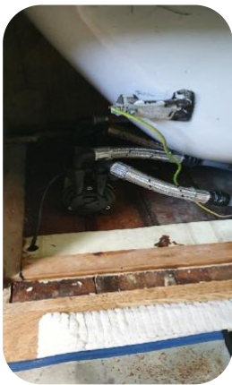
New flexi hose & earth bonding installed
