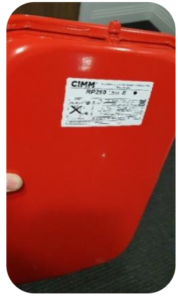
Installation of a new expansion vessel
