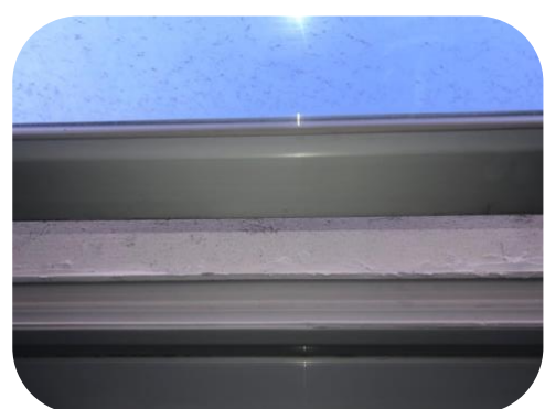
Installed new window rubber and window hinge
