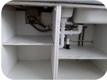
New sink trap & waste connectors
