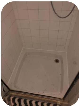
Sealed shower room
