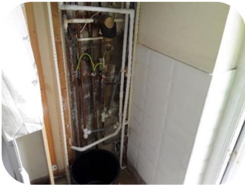
Installed new condensing pipe
