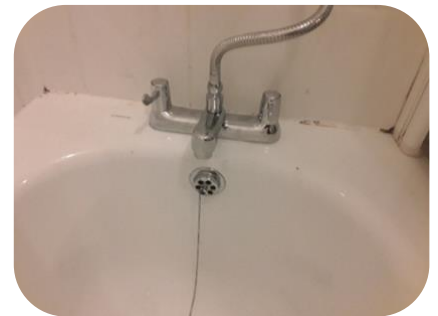
New mixer tap installed
