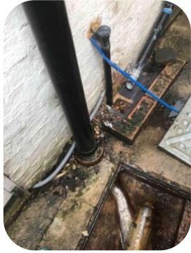
Cleaning drains following removal waste
