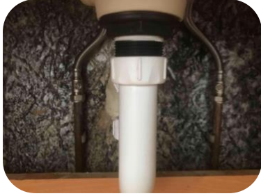
New waste pipe installed
