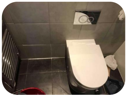
New toilet installation
