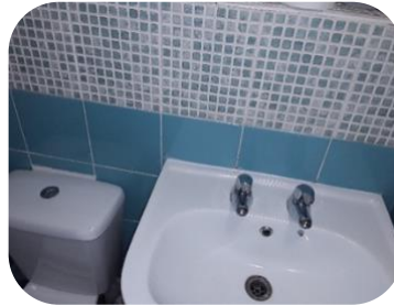
New sink & toilet installed
