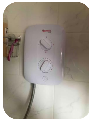
Installed a new shower
