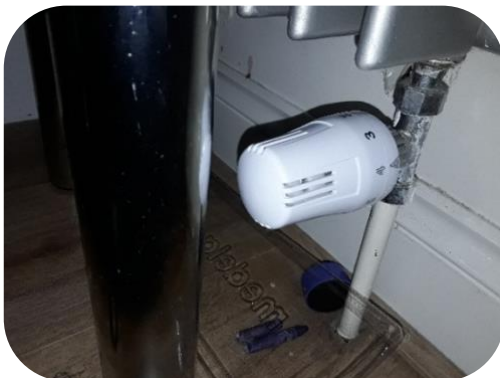
Installed new PRV valve
