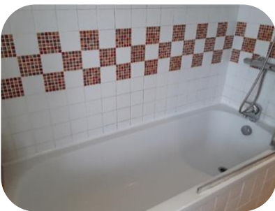
Installed new bath, tiling and sealed
