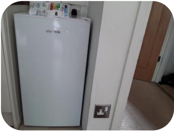
Installed 50cm wide fridge, with new power point
