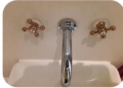
New mixer taps installed
