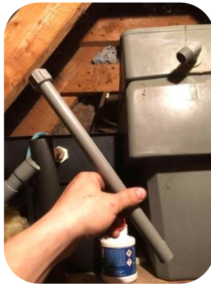
The overflow pipe being installed
