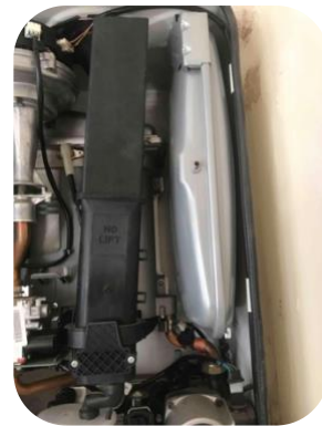
New boiler being tested during installation
