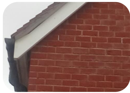
New lead flashing installed
