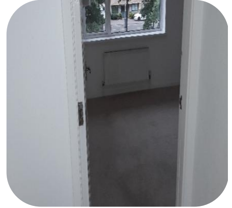
Installed new carpet & new PVC window
